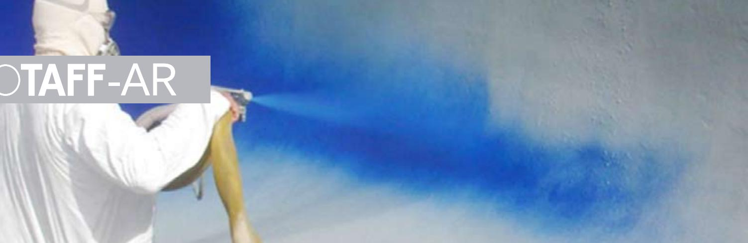
Hot Polyurea EUROT AFF AR is an ideal polyurea for indoor and outdoor coatings in industrial and commercial sectors. It retains no significant electric charging and therefore it is recommended for both flooring and coatings in electronic laboratories, white rooms, operating theatres or offices with
