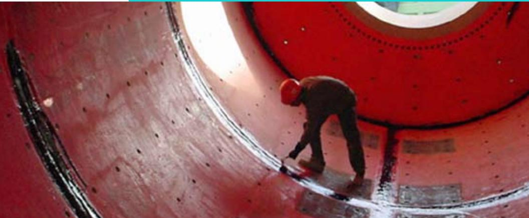
Due to the performance of polyurea against water and corrosion, together with its properties of potability, duration, resistance, drying and finish, it can be applied in numerous types of industries: petrochemicals, recycling plants, fish farms, filter systems, shipyards, agro-food industries, etc.
