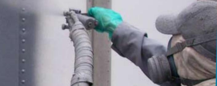
Due to its high resistance, elasticity and adaptability to all kinds of surfaces, polyurea is used in transport as a protective coating for loading bays, floors and side walls of lorries, vans, pick-ups or means of shipping transport.
