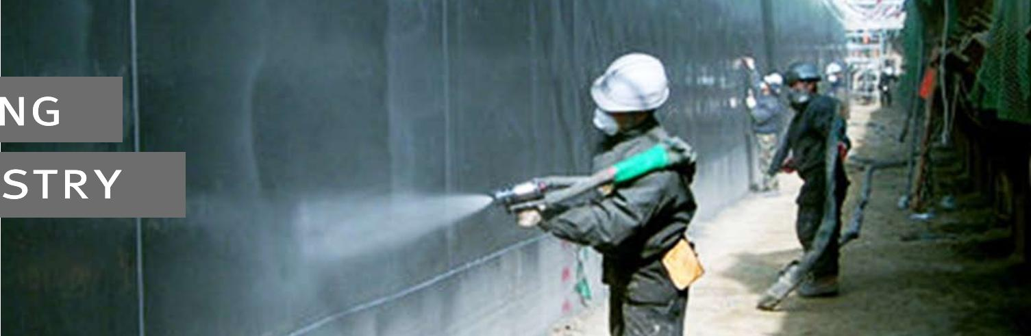
In the mining industry, polyurea is applied to: coating metal walls, floors and roofs/decks; protecting steel structures, tanks, pipelines and clarifiers; coating chutes, silos, classifiers and gridirons; protecting rollers and straps; coating for the protection of equipment and vehicle loading areas; coating evaporation pools to prevent pollution filtering into the land.
