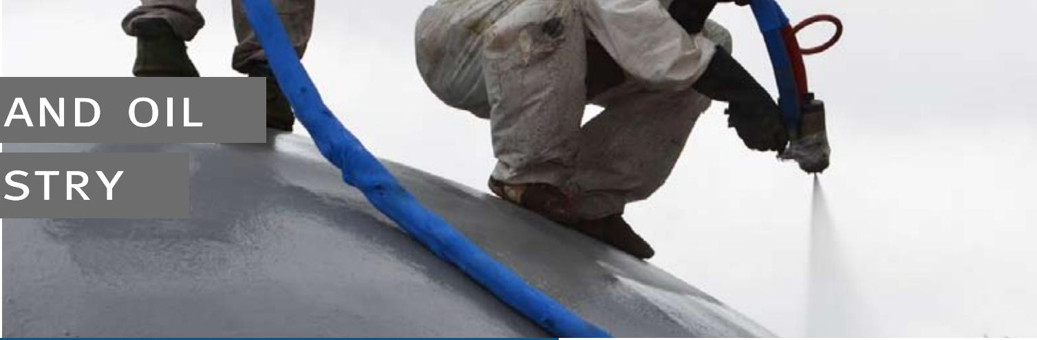
Polyurea is applied to the following in the gas and oil industry: protecting steel and concrete tanks; encapsulation of underground or overland pipelines; coating secondary retention containers to prevent spillage; coating evaporation pools to prevent pollution leaks into the land and for making corrosion-resistant floors, walls and roofs.
