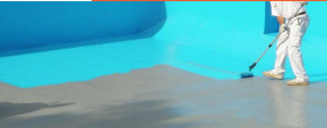
Cold polyurea EUROTAFF 300 is a polyurea that is stable against ultraviolet radiations. It is mainly used at domestic level or for small jobs. It is applied manually by rubber trowel or roller. Its drying time is slightly longer than that of hot polyurea.
