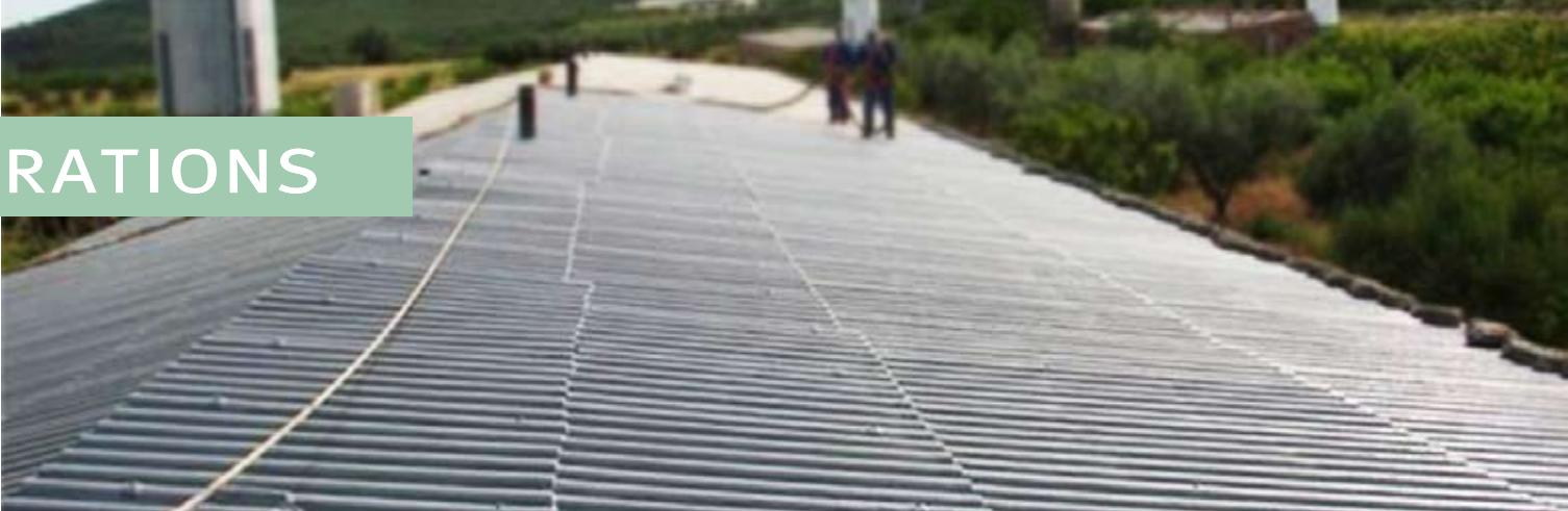
In the alteration sector, polyurea is applied as follows: waterproofing roofs, terraces, balconies and cantilevers; encapsulation of galvanized metal, metal sheeting, zinc, pre-lacquered and fibre cement roofs; protecting asphalt fabrics in bad condition and reproducing building and ornamental façade elements.
